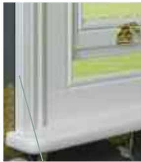
Slim Box Sash usually finishes flush with plaster work.
